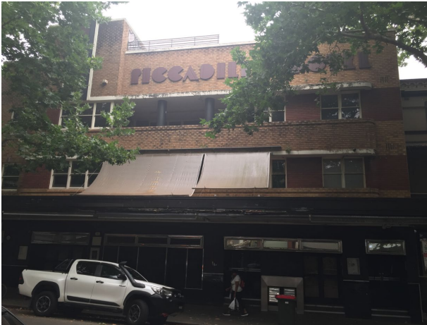
Figure 148 – Views directly in front of the subject site.
